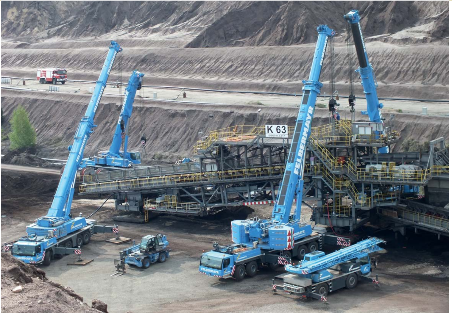
The renovation of the existing coal conveyor system meant the drive station had to be turned through 60 degrees.
