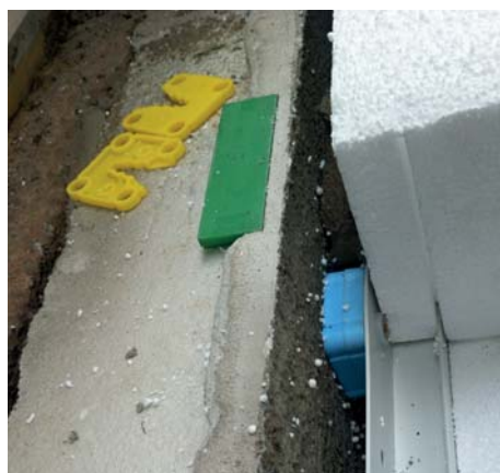
The Capatect PS thermal panels are suspended from slots in the rail system.
