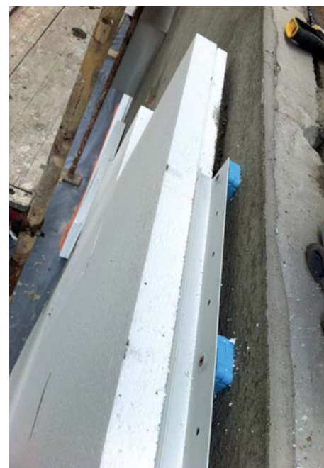
The Capatect rail system meant uneven and problematic areas could be concealed and a completely flat surface obtained.
