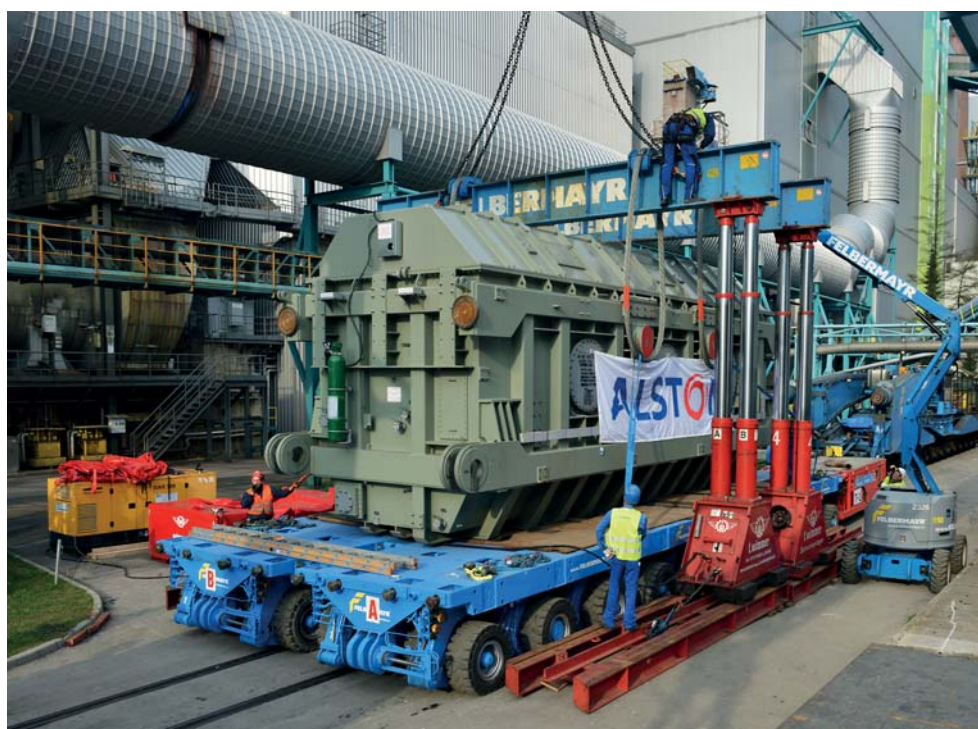
Personnel from Felbermayr's Wimmer subsidiary transferred the unit from the rail low-loader to the SPMT (Self Propelled Modular Transporter).
